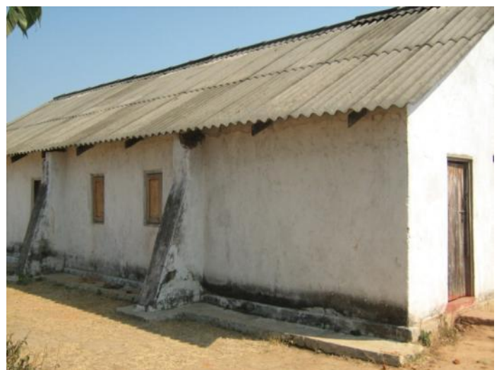
SDA Mwense Building
