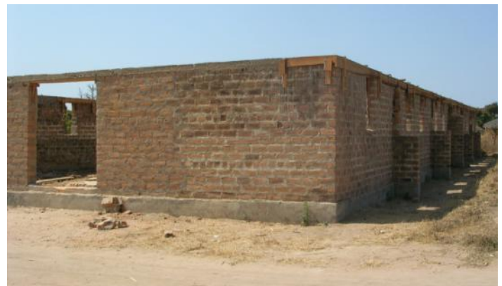
New building, in progress
