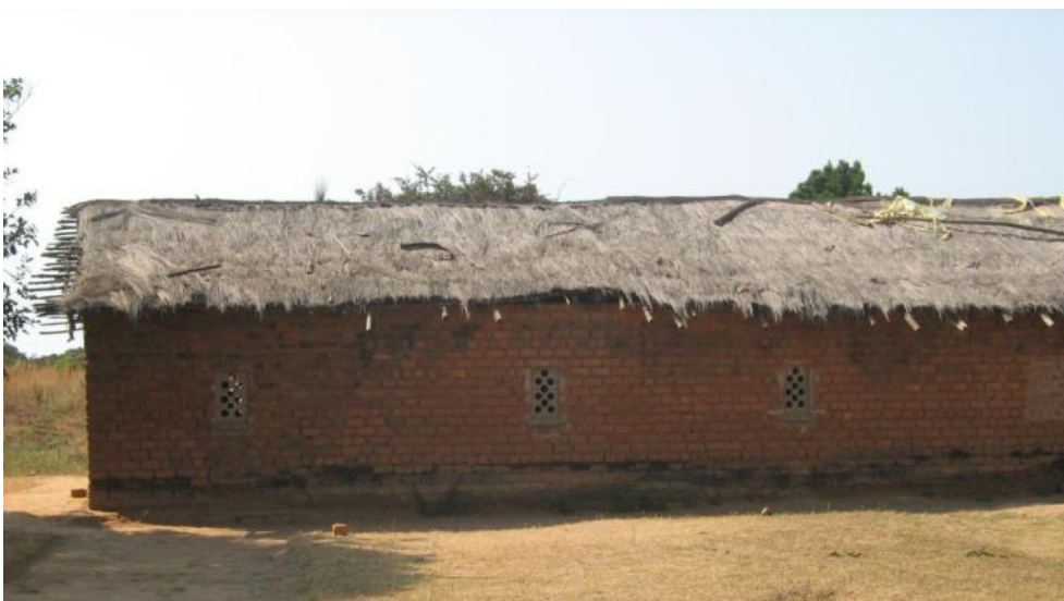
Church of God Chalwe's Building
